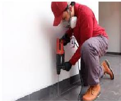
Post - Construction Termite Treatment
