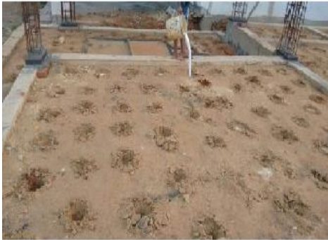
Pre - Construction Termite Treatment
